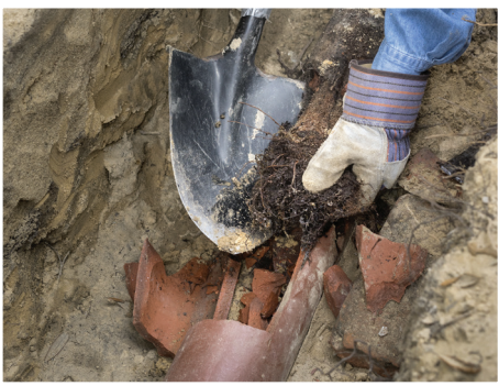
Plumber making repairs on private lateral
